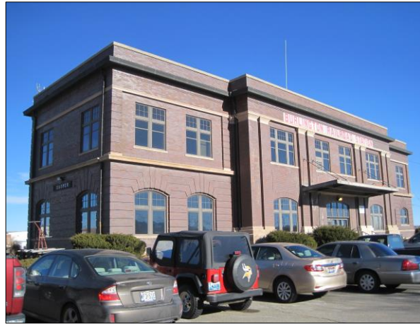
1916 Chicago, Burlington & Quincy Depot, 360 N. Wolcott St.
