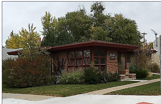
c1949 Contemporary Style office, 843 S. Center St.
