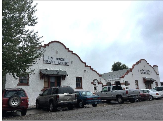
c1920 Multi-Unit building, 139 N. Grant St.
