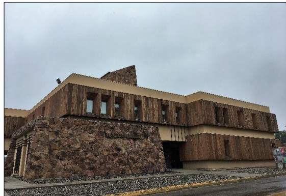
1973 Brutalist building, 167 S Conwell St.
