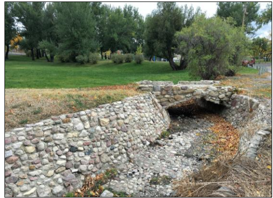
1930s Washington Park Grounds, 951 S. Jefferson St.
